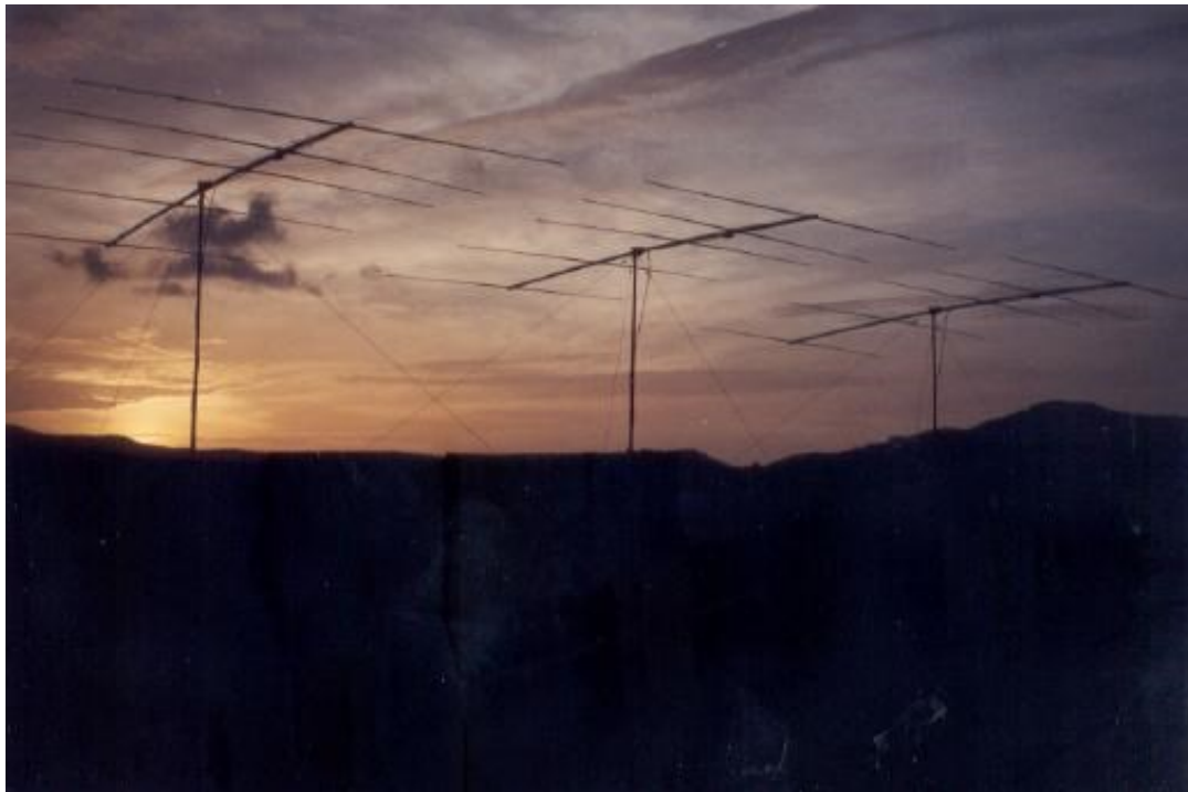
Figure 1.10. Part of the array composed of eight Yagi-Uda antenna of the CSR at St. Croix, USVI [Cornell University, http://landau.geo.cornell.edu/ ].
