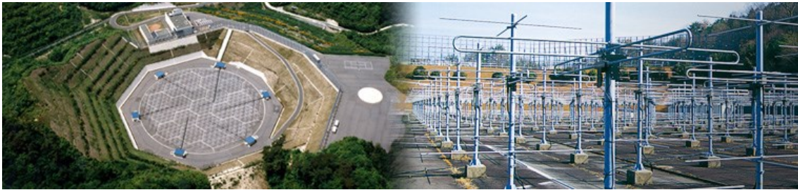
Figure 1.11. Overview and the antenna array of MU radar at Shigaraki, Shiga, Japan [Research Institute of Sustainable Humanosphere (RISH), Kyoto University, http://www.rish.kyoto-u.ac.jp/mu/radar.html ].
